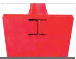
For robustness the steel beam is set into the floor plate and welded on both sides
